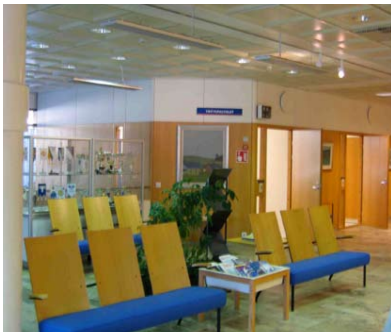
Figure 2. Privacy solution in bank branch waiting area. The speakers are hanging from the ceiling and are adjusted directly above the seating rows.
